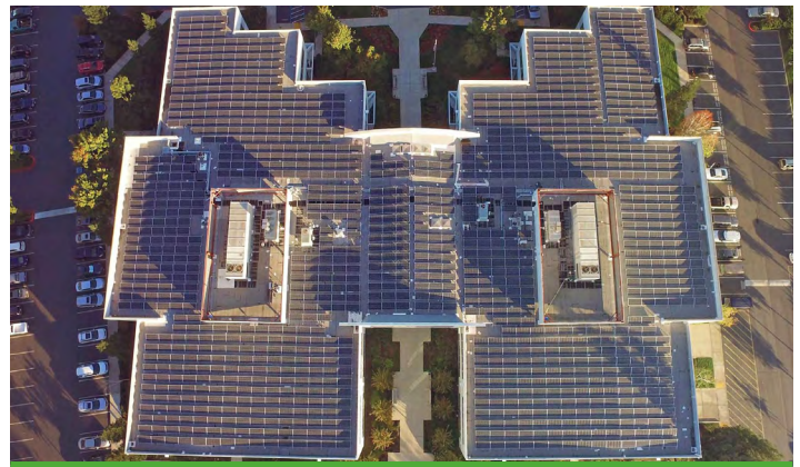
Aerial view of solar panels on the rooftop of a building in Rancho Cordova, California. Photo credit Michele Parry.
